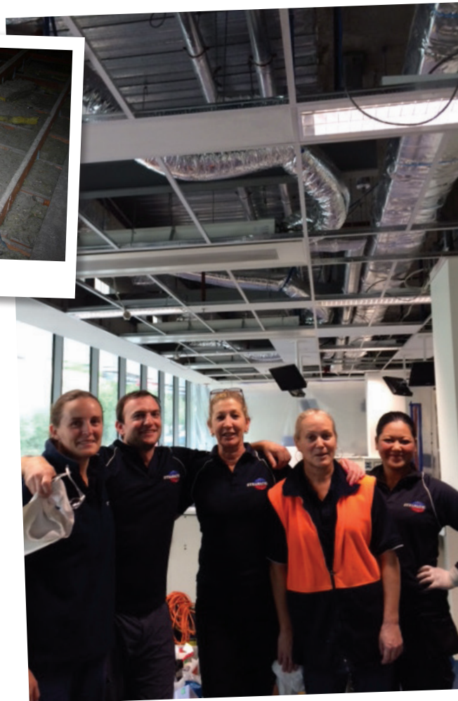
The Steamatic team on the job at the Box Hill Hospital.
